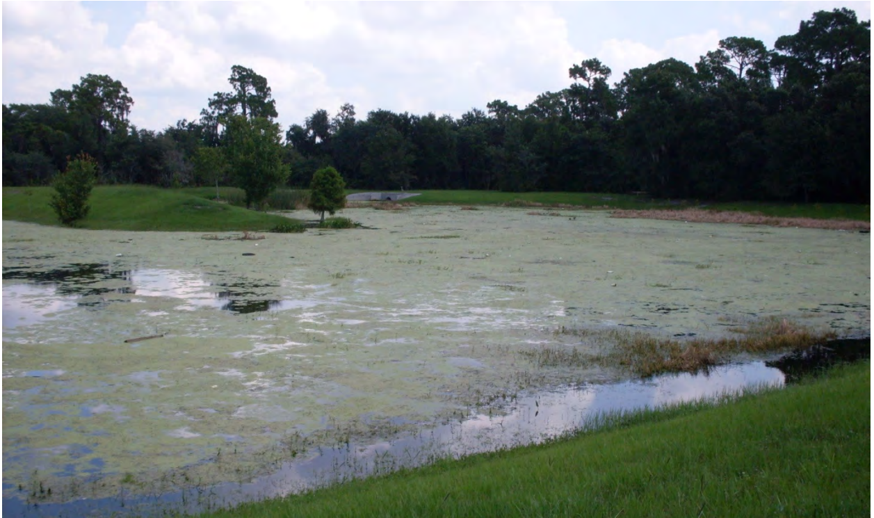
Photo 4-15. Lake Jessie stormwater treatment project at Derby Avenue.
