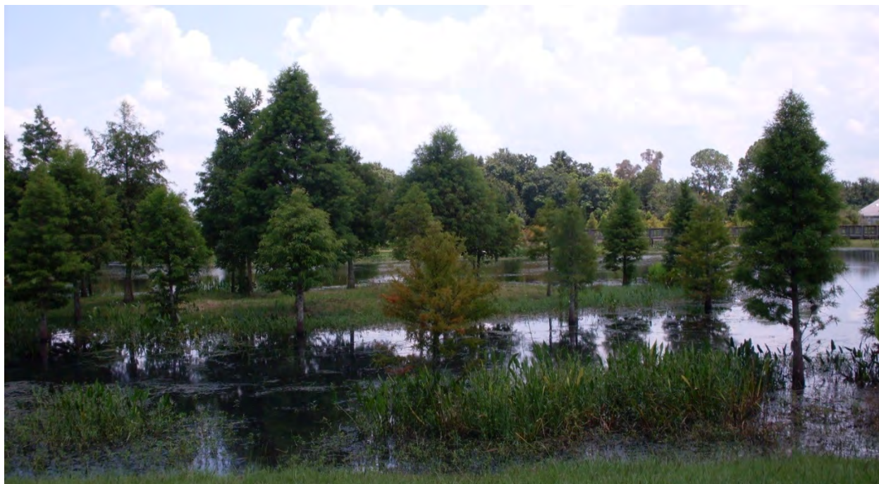
Photo 4-12. South Lake Howard wet detention stormwater treatment project.
