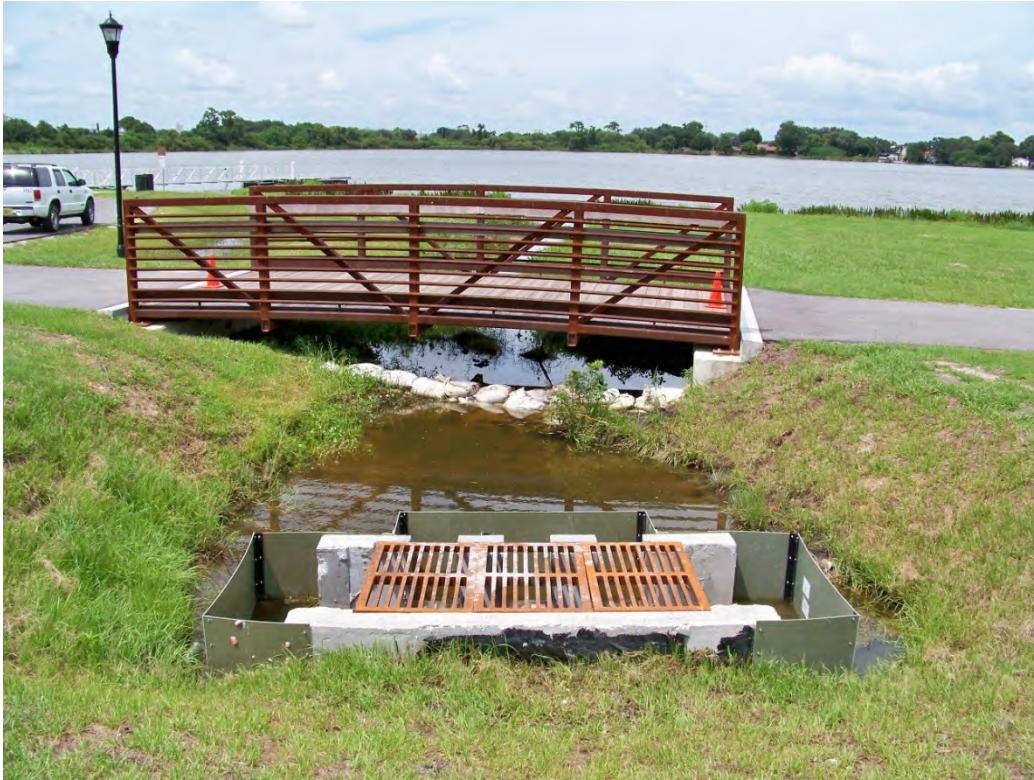
Photo 4-1. Water control structure at southern end of Lake Blue.
