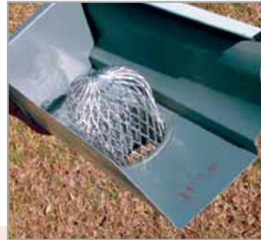
A window screen placed over the barrel opening (left) or a gutter strainer placed in the downspout opening (right) will keep leaves and other debris out of the rain barrel.
