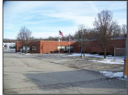
Street Department Facility on Nelson Avenue
