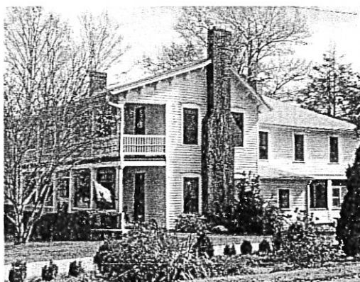
Figure 1: The two chimneys that need repair are the two exterior, end chimneys which are situated at the gable ends of the main/front block of the house.
