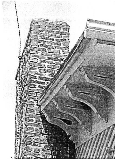
Figure 3: The tops of the chimneys above the roofline are unstable, so it is necessary to dismantle and re-lay the top courses of the chimneys.
