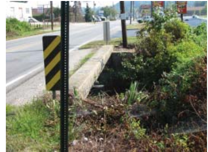
Allens Creek Bridge without railing and sidewalk.
