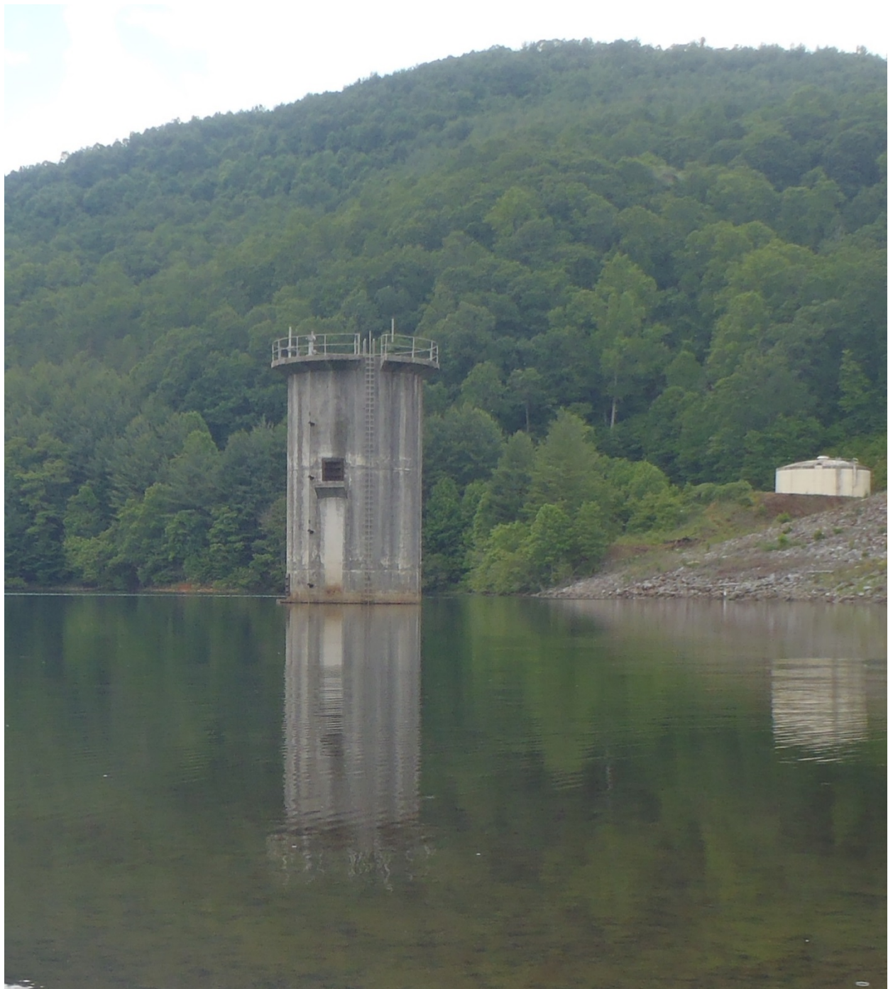
Figure 7 - Available Intake Gate at 3,195'
