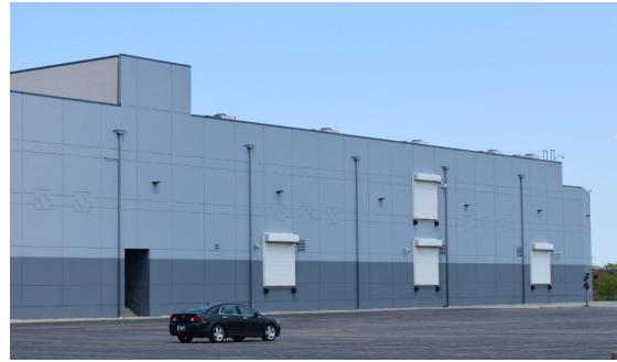
2-level data floor, Cyxtera, Elk Grove Village, IL
