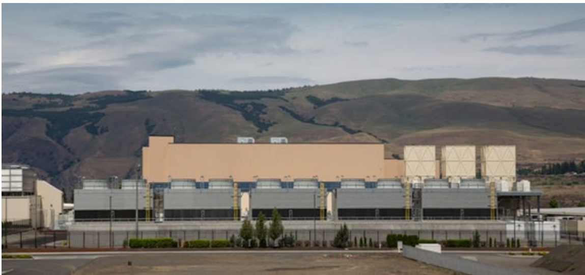
Facebook data center campus, The Dalles, OR
