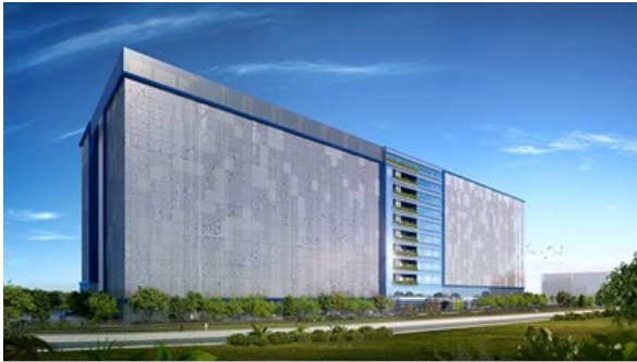
11 level data center, Google, Singapore
