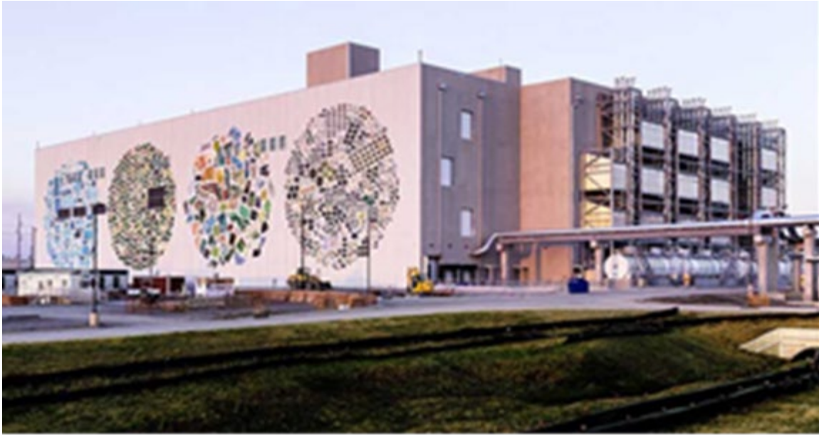
Facebook data center campus, Pryor, OK
