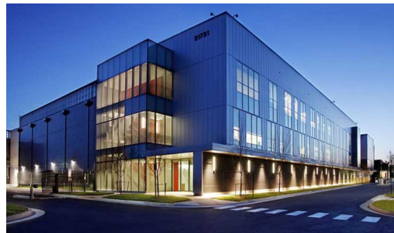
3-level data floor, Equinix, Ashburn, VA
