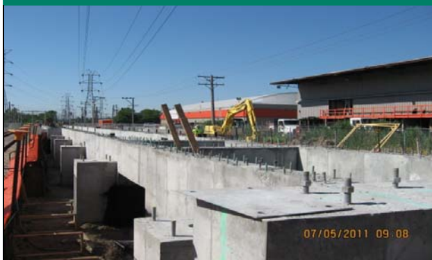
Foundation walls are complete on the South Station house
