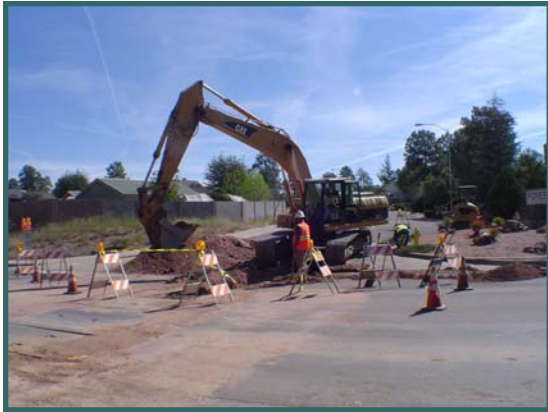
“Line E” Construction
