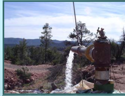
Groundwater being pumped from a TOP Well
