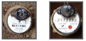
If the red dial or black triangle is spinning that means water is passing through the meter and you should check around your home for signs of a leak. For a more detailed explanation please see our brochure <u>"How to Read Your</u> <u>Water Meter"</u>.
