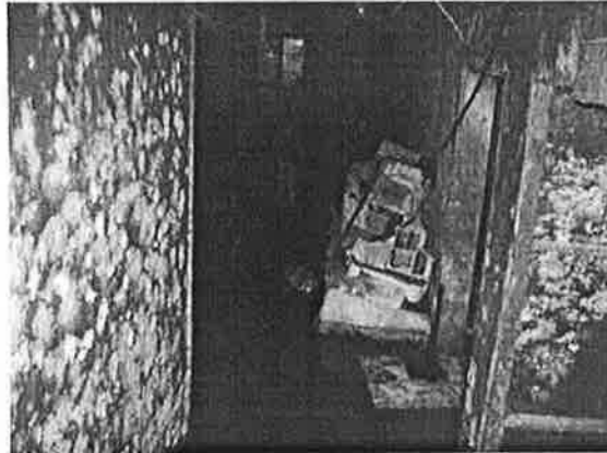
Sewage water accumulation and possible mold accumulation in basement (TS, 06/04/14)
