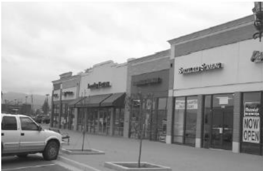
Figure 12-13: Example of Appropriate Use of Wall Offsets, Material Change, and Roof Line Changes
