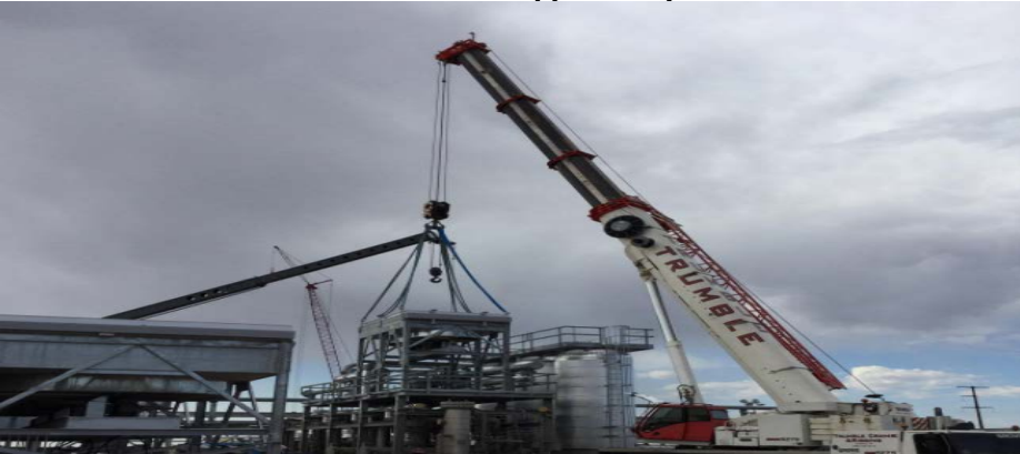
Installing Dehydrator
