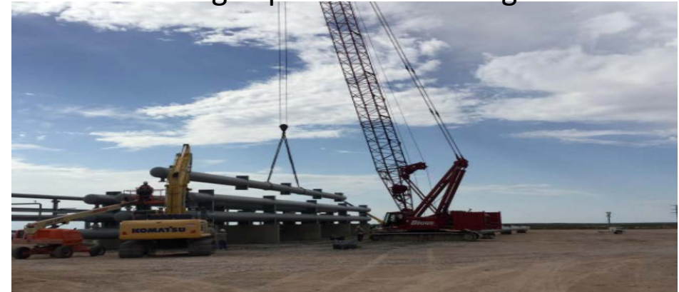
Installing Top Headers on Slug Catcher
