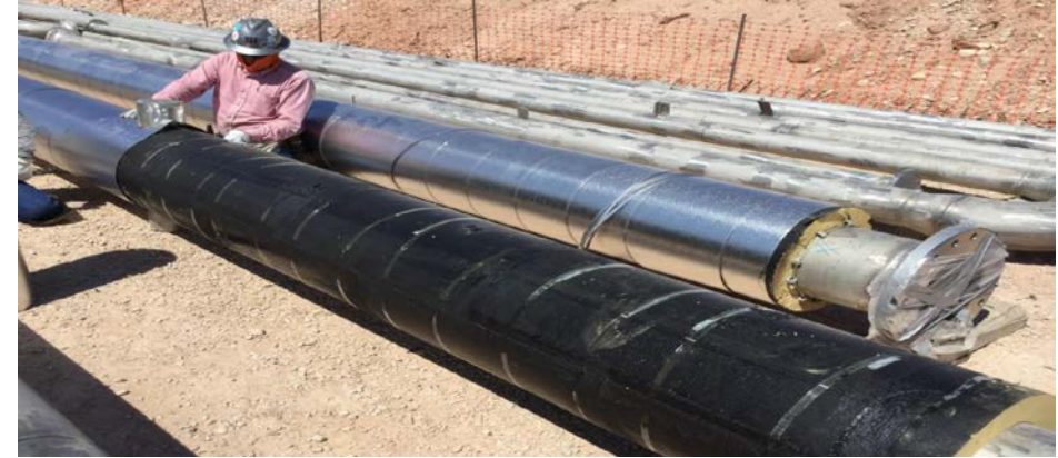
Insulating Cryogenic Area Pipe
