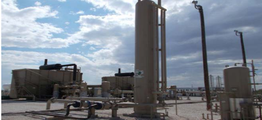
Pecos Dehydrator and Compressors
