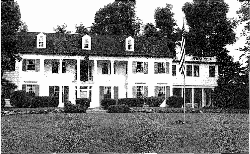
The Rollmans' home was completed in April 1928.
