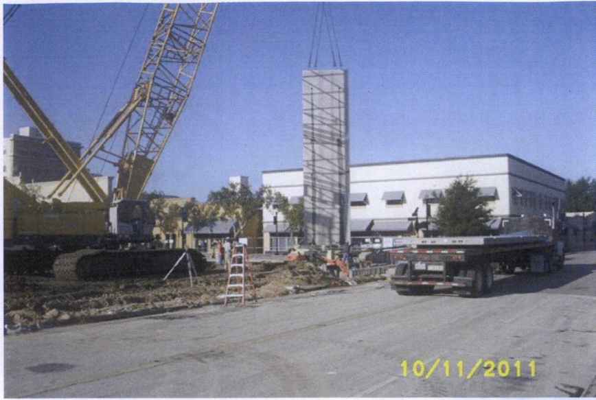
First panel put in place October 11, 2011
