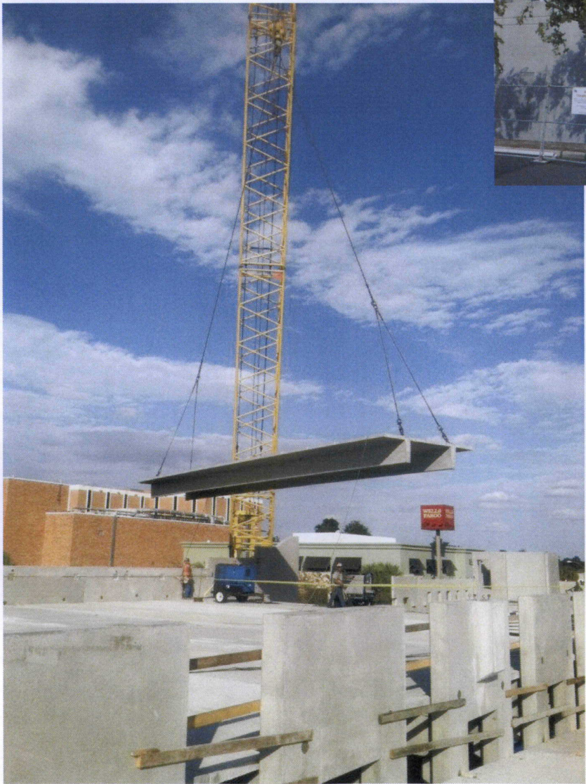
Last panel put in place November 1, 2011
