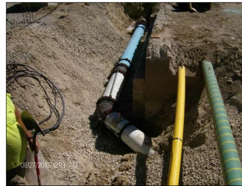
After: Water main repaired by Water Distribution Employees at Swindler's on 8/28/10.
