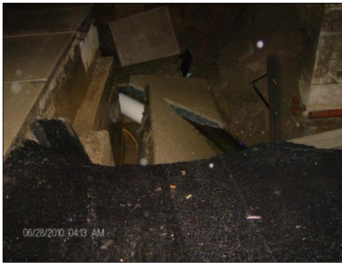
Before: Water main damaged by flood sinkhole on 6/28/10 at 2 a.m.
