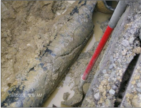
Broken water main on Old SR 73 at PC Connection
