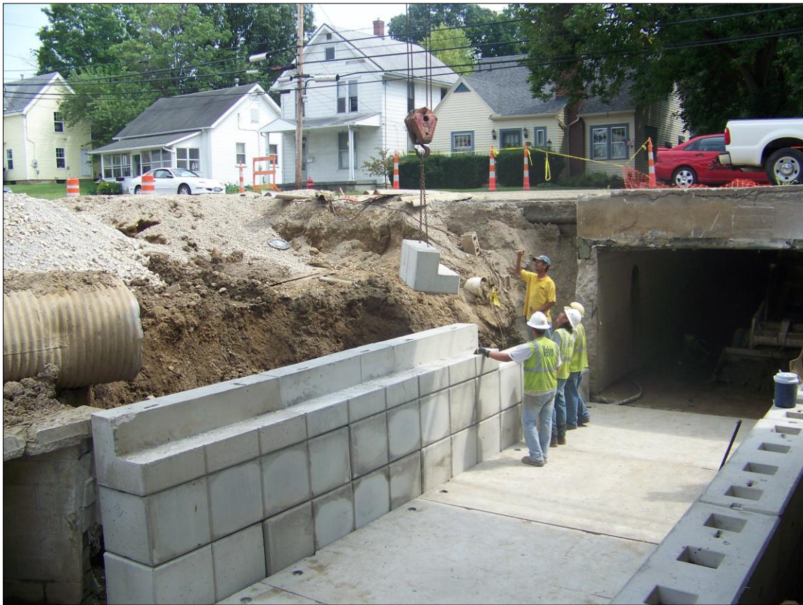
Storm Water Project at Swindler's – 321 West Locust Street
