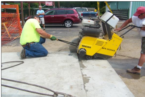
Cutting Concrete Slab for Storm Culvert Project
