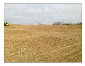
Phase 4 is roughly a three-acre site that is situated on the southeast side of the old capped landfill. It is expected that by fall of 2015 we will start waste placement in Phase 4. This design of the vertical expansion allows the city to recapture airspace above the old clay-lined fill without increasing the overall footprint of the total landfill. The total vertical expansion plan of five phases should provide the city an extended airspace life of twelve-plus years.
