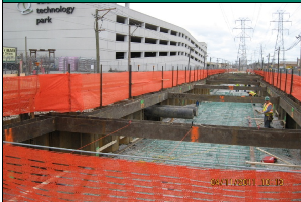
Preparation work for concrete slab in utility tunnel
