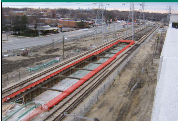
Aerial view of utility tunnel
