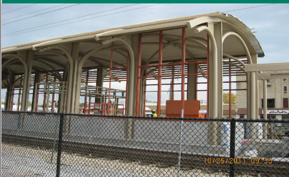
Aluminum Curtain Wall and Permanent Site Fencing at North Station House
