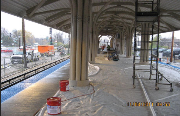
Blue Tactile Edge Tile and Painting at South Station House
