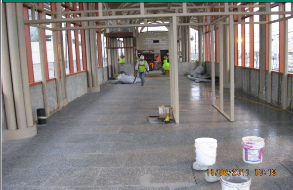
Granite Flooring at North Station House
