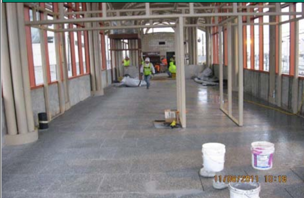
Granite Flooring at North Station House
