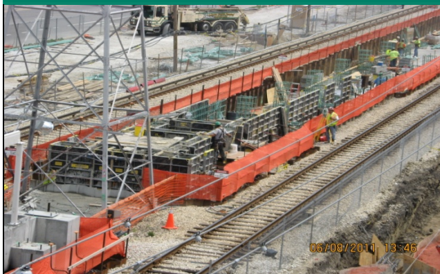
Foundation walls have begun at the South Station
