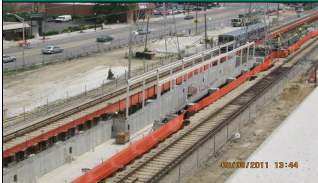
The walkway at the North Station is taking shape
