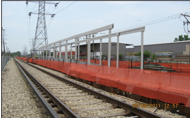
Structural steel erection has begun!
