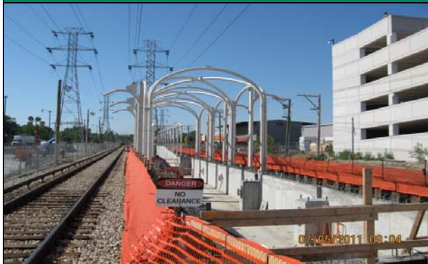
The North Station house is taking shape
