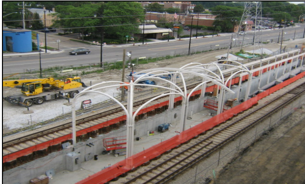
Structural Steel columns and arches at North Station House
