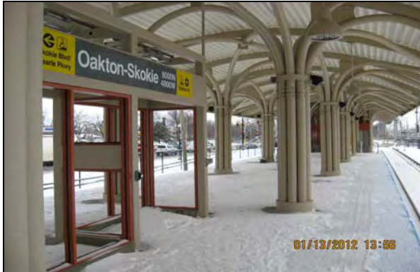
Finishes at windbreak on the platform
