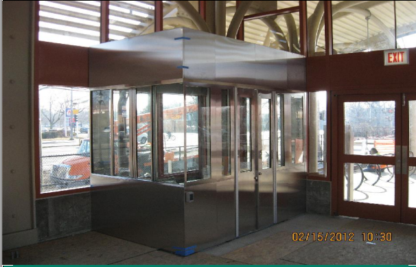
The stainless panels, glass and doors at the South Station House customer assistance kiosk
