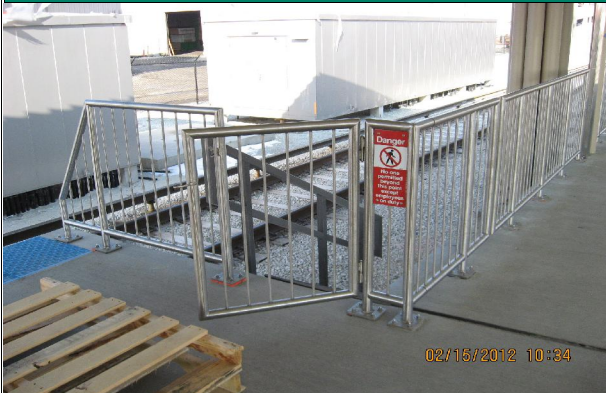
Guardrails and access stair installation on the platform
