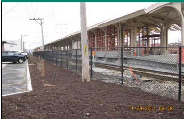
Newly installed landscaping and site fencing
