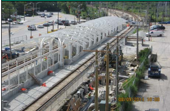
The South Station House is progressing
