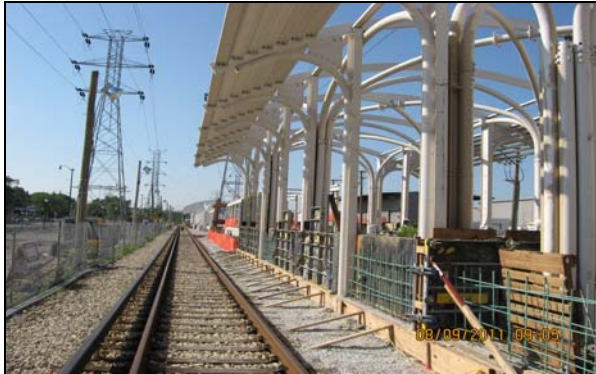
Architectural walls are being installed at the North Station House
