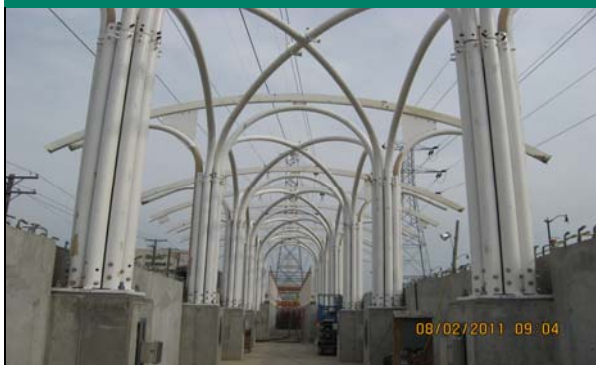
Structural arches and columns on the South Station House
