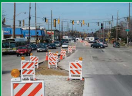
Pre-Stage work northbound Skokie Boulevard from Foster Avenue
