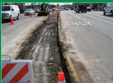
Temporary pavement work on Skokie Boulevard near Golf Road
