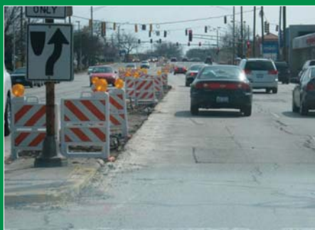
Pre-Stage work on Skokie Boulevard south of Golf Road
