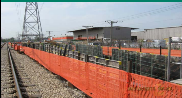
Foundation walls have begun
