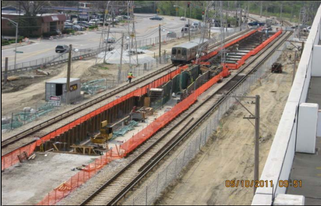
Tunnel excavation is complete!
