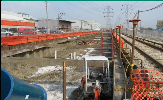
Final phases of underground plumbing installation
