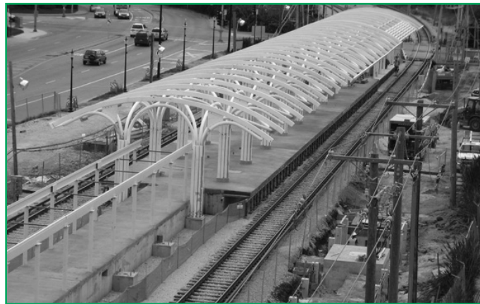
Current view looking south of the CTA Yellow Line Oakton Station in Downtown Skokie.
