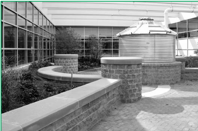
Water cistern located in one of two internal courtyards at the Skokie Police Headquarters. The cistern harvests rainwater from the roof to irrigate landscaping on the property.
