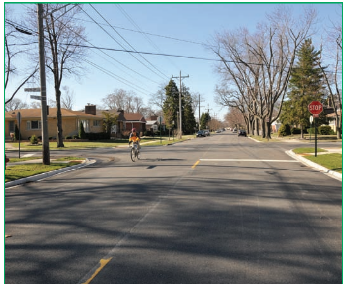
East Prairie Road Resurfacing
