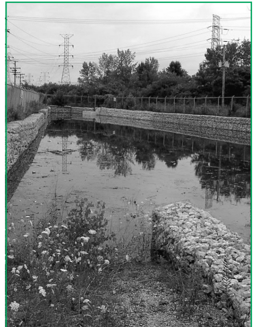
Shown above: Gabion Pond on Oakton Street in Downtown Skokie. Depressed landscaped areas like Gabion Pond are used to detain stormwater runoff during heavy rainstorms. The ponds fill with excess water and drain into the combined sewer system at a rate that reduces the chance of sewer surcharge.
