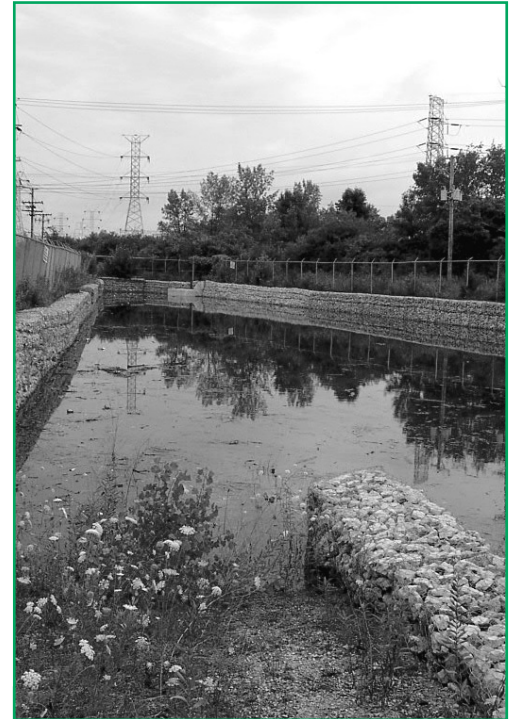
Shown above: Gabion Pond on Oakton Street in Downtown Skokie. Depressed landscaped areas like Gabion Pond are used to detain stormwater runoff during heavy rainstorms. The ponds fill with excess water and drain into the combined sewer system at a rate that reduces the chance of sewer surcharge.
