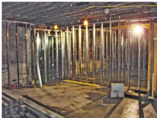
Work Progressing - Administration Office, Library in Basement
