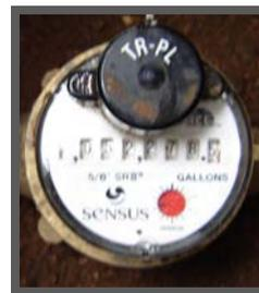
If the red dial or black triangle is spinning that means water is passing through the meter and you should check around your home for signs of a leak. For a more detailed explanation please see our brochure [“How to Read Your Water Meter”](#).
