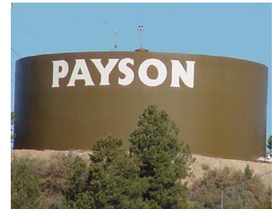
Payson's signature water tank, as seen from Highway 87 when entering Payson.
