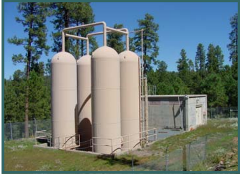
C.C. Cragin Pump Station
