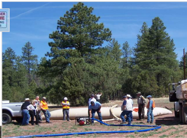
Surplus Military "Pillow Tanks" were purchased by Gila County and installed by County Public Works personnel.
