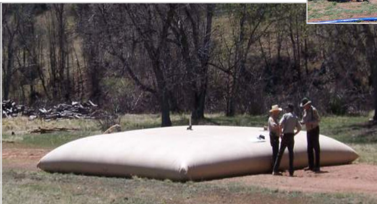
Surplus Military "Pillow Tanks" were purchased by Gila County and installed by County Public Works personnel.
