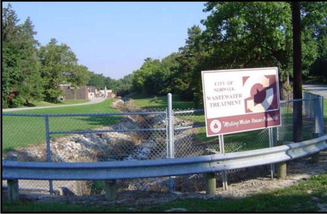
Site of the Norwalk Wastewater Treatment Plant off of Lais Road.
