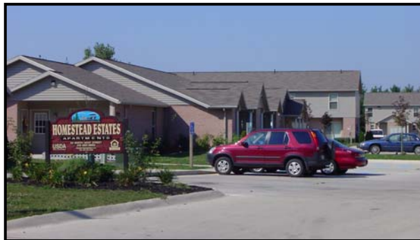
Newer subsidized housing in Norwalk: Homestead Estates on N. West Street.
