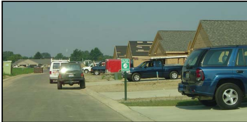
New homes under construction at Hunter's Glen
