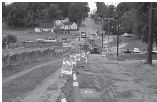
Church Street Improvement Project, September 2009
