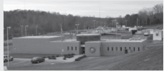
Rocky River Wastewater Treatment Plant
