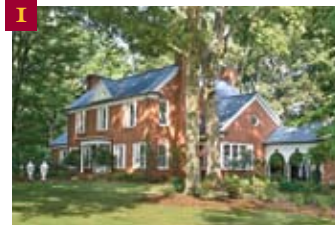
I The J.A. Stewart House (ca. 1896) 832 North Main Street 5400 sq. ft. home to the founder of the Mooresville Cooperative Creamery.
