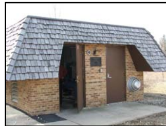
Well No. 2 Well House Building
