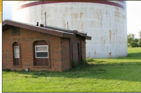
Well No. 5 Well House Building in foreground, 2.5 MG Ground Storage Tank in the background
