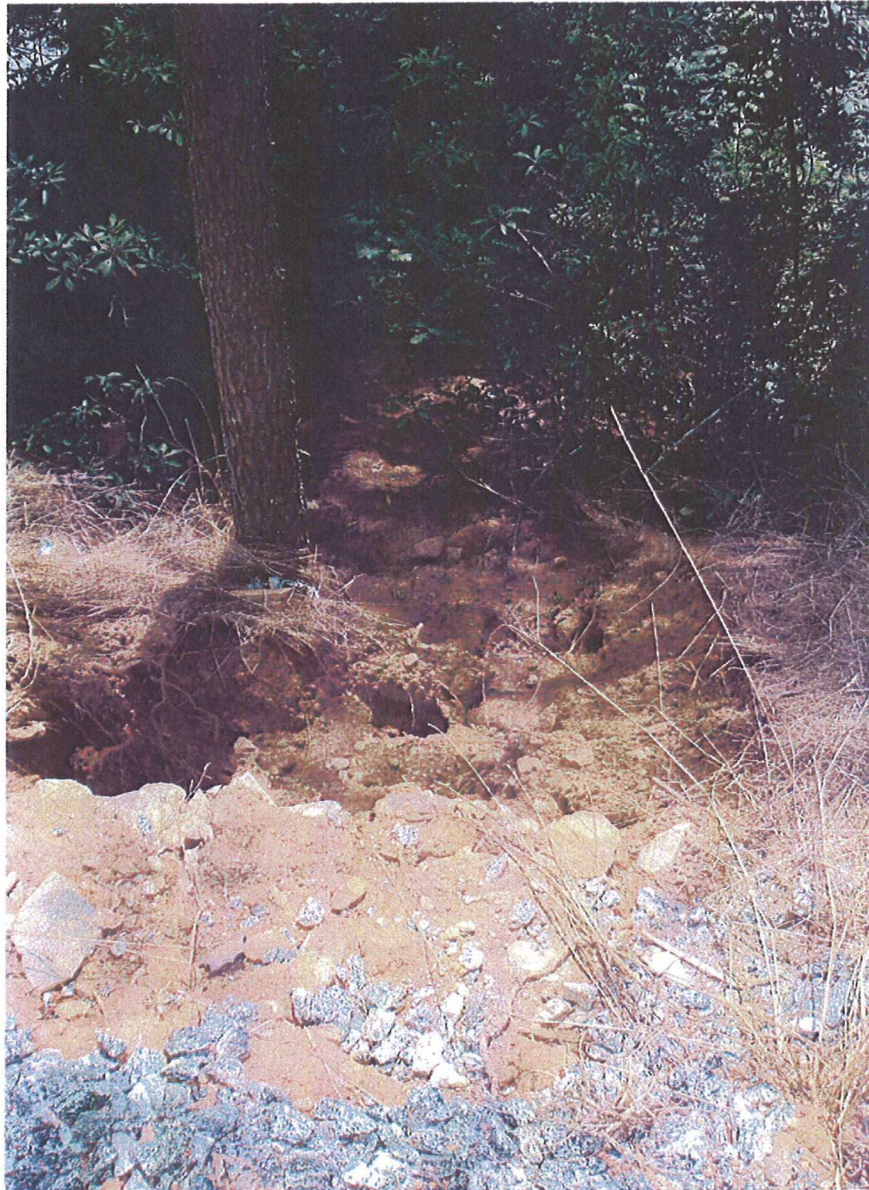
Erosion from well flushing; repair, and seed
