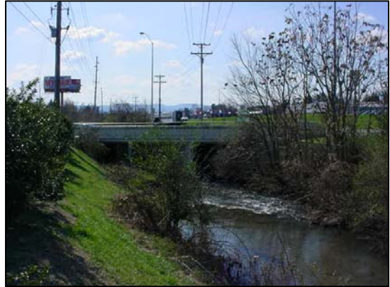
Anderson Street Bridge over Little Creek
