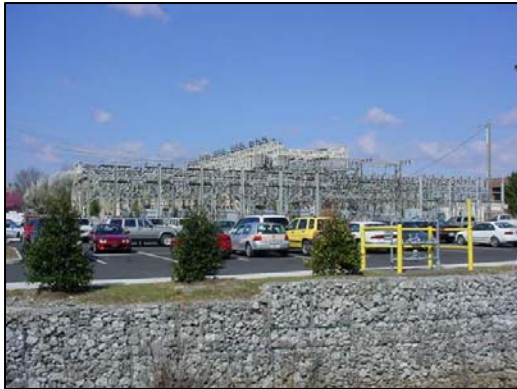
New Parking Lot
